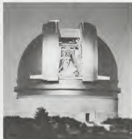
Hale reflector dome with shutter open
